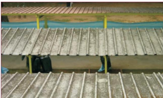
Asbestos roof sheets (front & centre) and zinc roof sheets (back)
